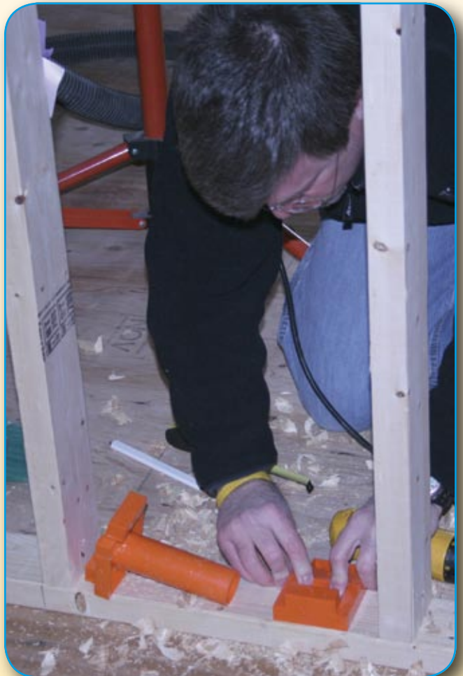
A worker installs a mounting bracket.
