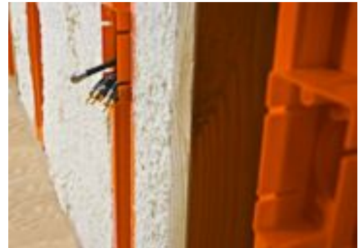
The eXapath system shown in sprayfoam insulation
